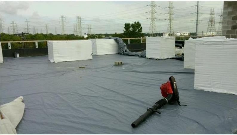
An additional stage of completely covering and protecting the installed insulation board required the use of plastic sheathing before any spray foam could be applied. As always, the roofing surface needed to be clean, dry and stable.
