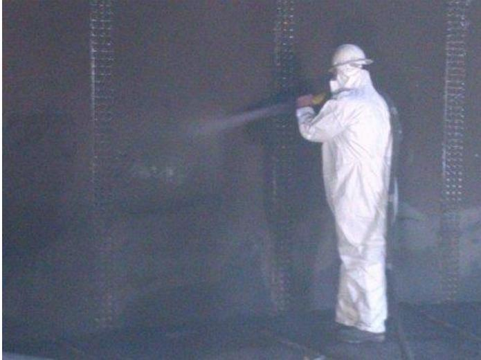
It was then time for the crew to apply 80 mils (2,032 microns) of Oak Ridge OR-70SS polyurea topcoat using a Graco Reactor E-XP2 plural component proportioner. “The main reason this coating system was chosen was for its excellent chemical and abrasion resistance properties. The polyurea can withstand the extreme conditions that exist inside of the tank,” explained Franklin.
