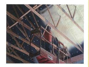
SAVING ENERGY AND KEEPING THE PRODUCE FRESH RELIES ON TOTAL ENCAPSULATION OF THE BUILDING'S INTERIOR, USING A MINIMUM OF TWO INCHES OF SPRAYED APPLIED 2 LB. DENSITY POLYURETHANE FOAM INSULATION TO WALLS AND UNDERSIDE OF THE ROOF DECK.
