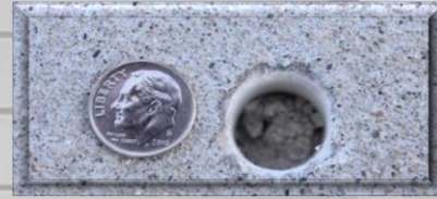
Foam injection uses fewer, smaller holes; only 5/8" in diameter.
