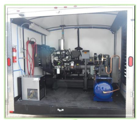
Air dryer will keep the humidity levels down within the air supply system.
